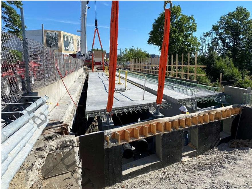
Figura 8. Sistema constructivo PBU (Fort Miller Company, 2016).
